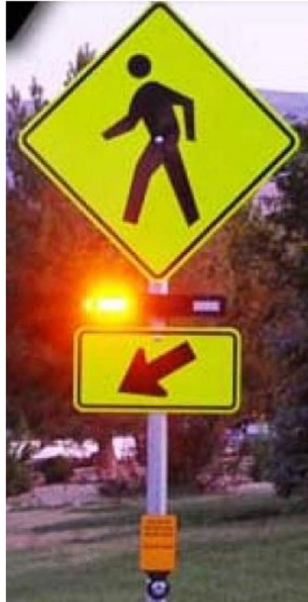
RFB uses irregular flash pattern similar to emergency flashers used on Police and emergency vehicles referred to as wig-wag or stutter flash pattern.
